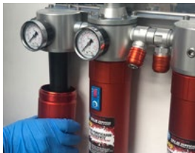
Unscrew lower section
