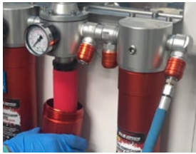
Unscrew lower section
